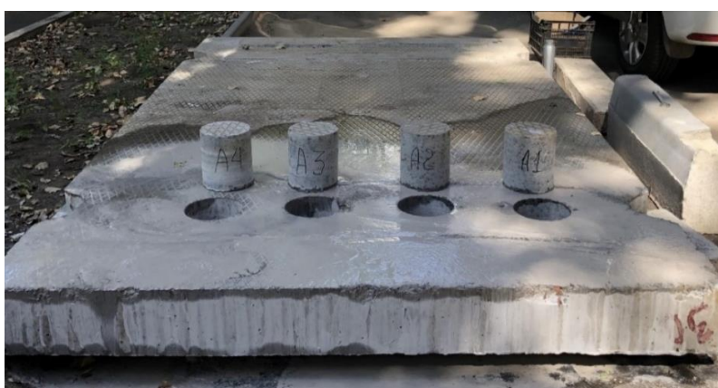
Figure 7. Drilled cores of the slab
